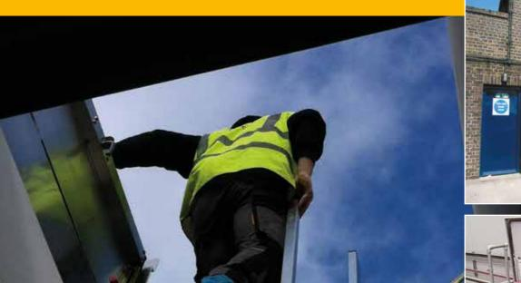
Manufactured in either aluminium or galvanised steel, our range of fixed vertical ladders are ideal for personnel access. These can be provided with a safety cage or guardrail if required to meet the relevant British Standards.
